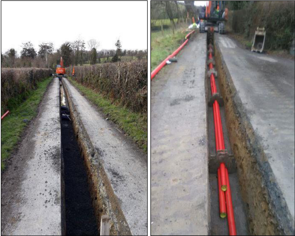
Plates 1 & 2: Typical Trench Construction (Note: Proposed works within public road network relate to road crossings)
